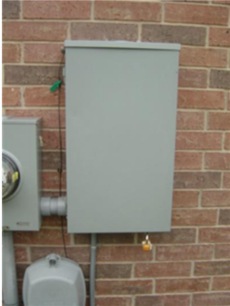
A. Picture 1 Locked main service panel
